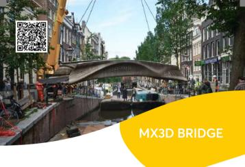
The MX3D bridge is a functional construction that will be used for crossing a canal, made of stainless steel from robots and 3D printing.
