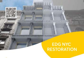
EDG NYC is an architectural firm that has developed a new digital sculpting method called "Modern Ornamental" to restore a building in New York City. The process uses 3D printing to produce complex molds for molding concrete structures
